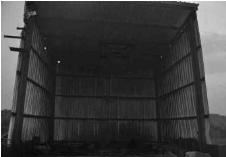
Water Arrangement at CHP Hooper
