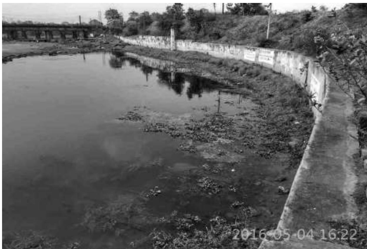
Toe wall and Embankment at Cluster IV
