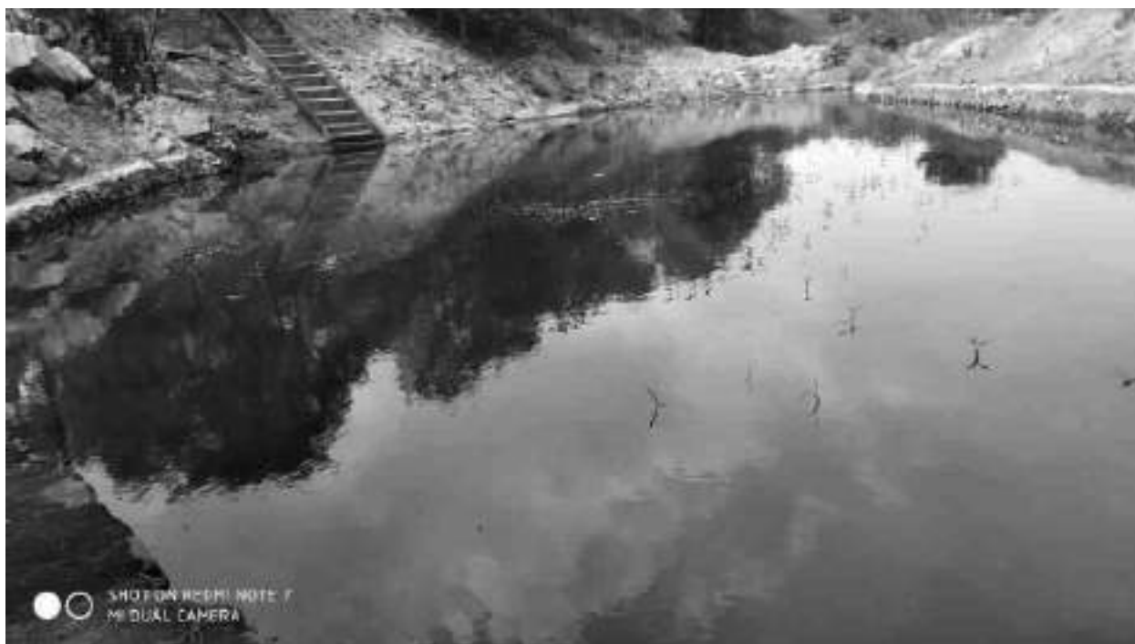
Rain Water Harvesting Pond at Green Park,Cluster-IV
